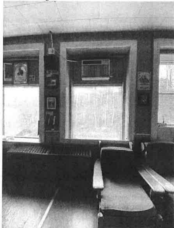
View of centered windows on front wall of Day Room with plywood infills and fixed window units replacing orig. double hung sash.
