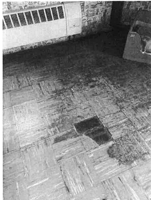
Vinyl composition tile (VCT) on floor is in poor condition in many locations. 9" square VCT typically contained asbestos & is considered a HAZMAT.
