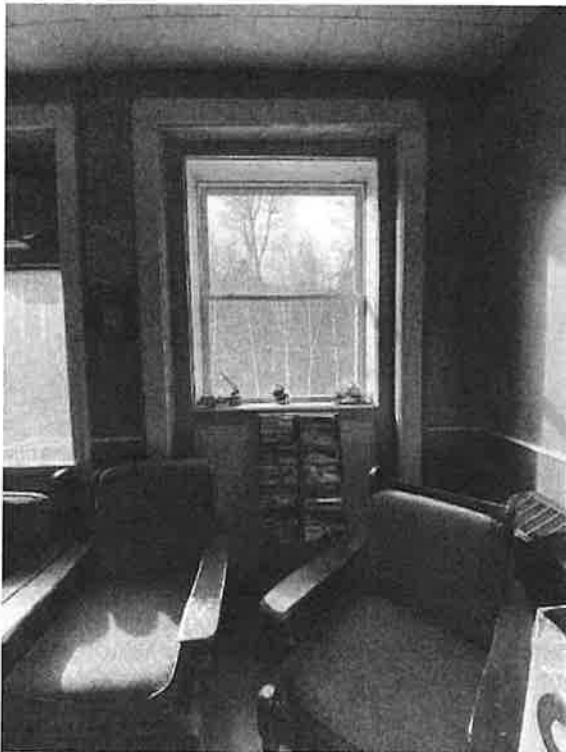
Detail view of orig. doorway opening to front balcony, now infilled with a small window unit.
