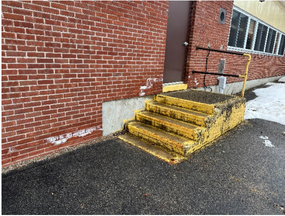
Figure 7 North Entrance Concrete Damage
