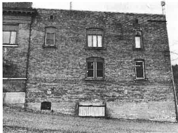
South elevation with altered window openings.
