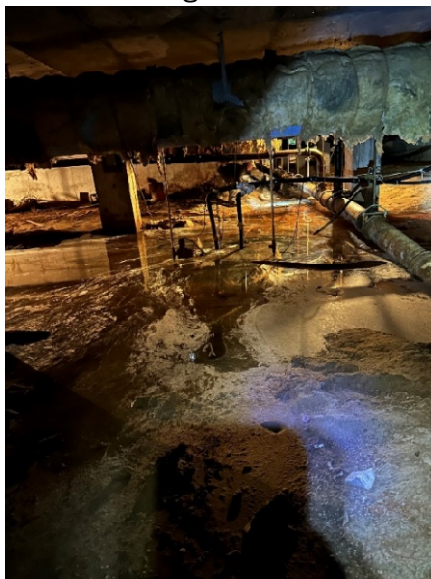
Figure 3 & Figure 4 Water Infiltration in Crawl Space
