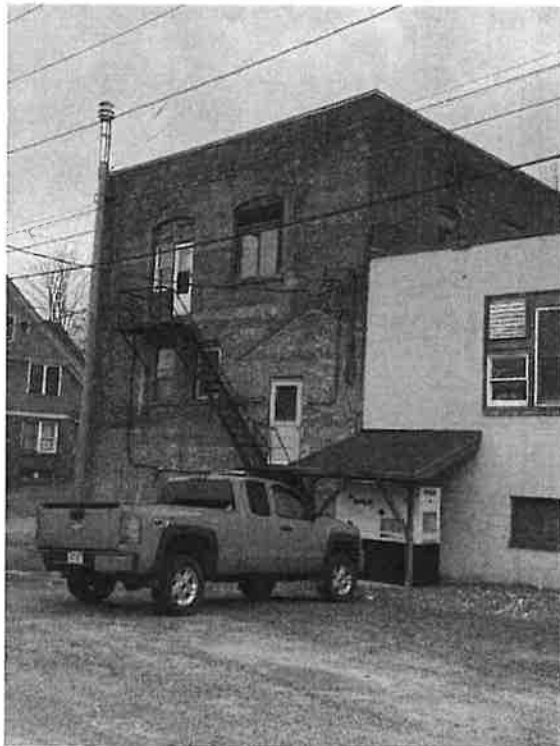
View of north elevation showing altered window openings and c.1960s CMU addition.
