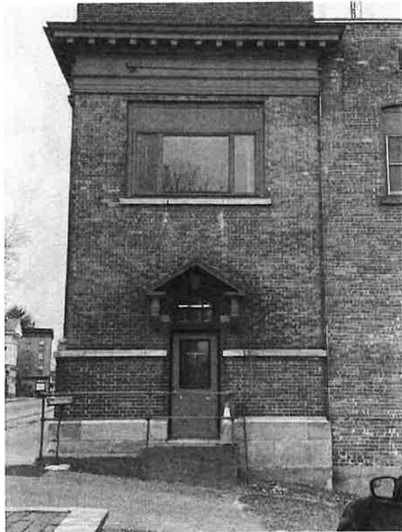
Original side entry with replacement door and framed down and altered 2 nd floor window.
