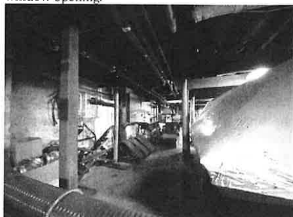
View of parged foundation wall on north side of basement with former window openings to crawl space of 1960s addition infilled with plywood.
