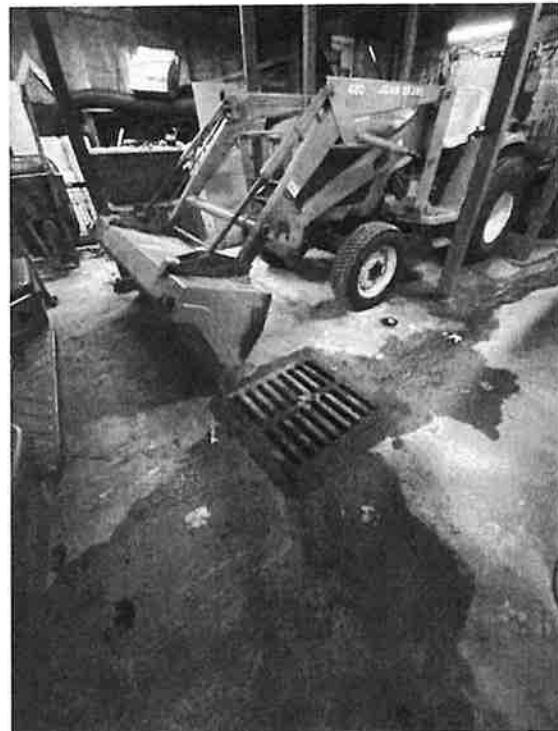
Large drainage grate positioned in center of basement floor for site water from rear yard.
